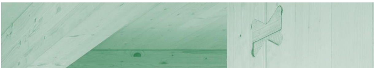
Figure 11: Fully wooden connections allow for disassembly, Collegium Academicum. Photo: Thilo Ross.
