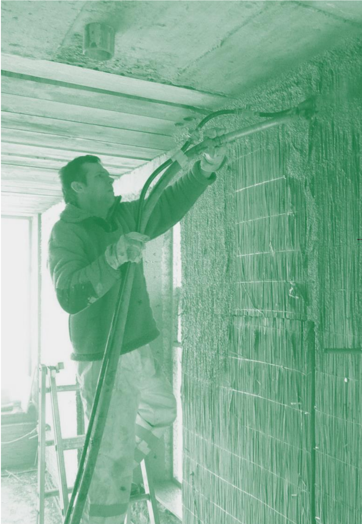
Figure 12: Bio-based interior finishes, Haus Rauch. Photo: Martin Rauch
