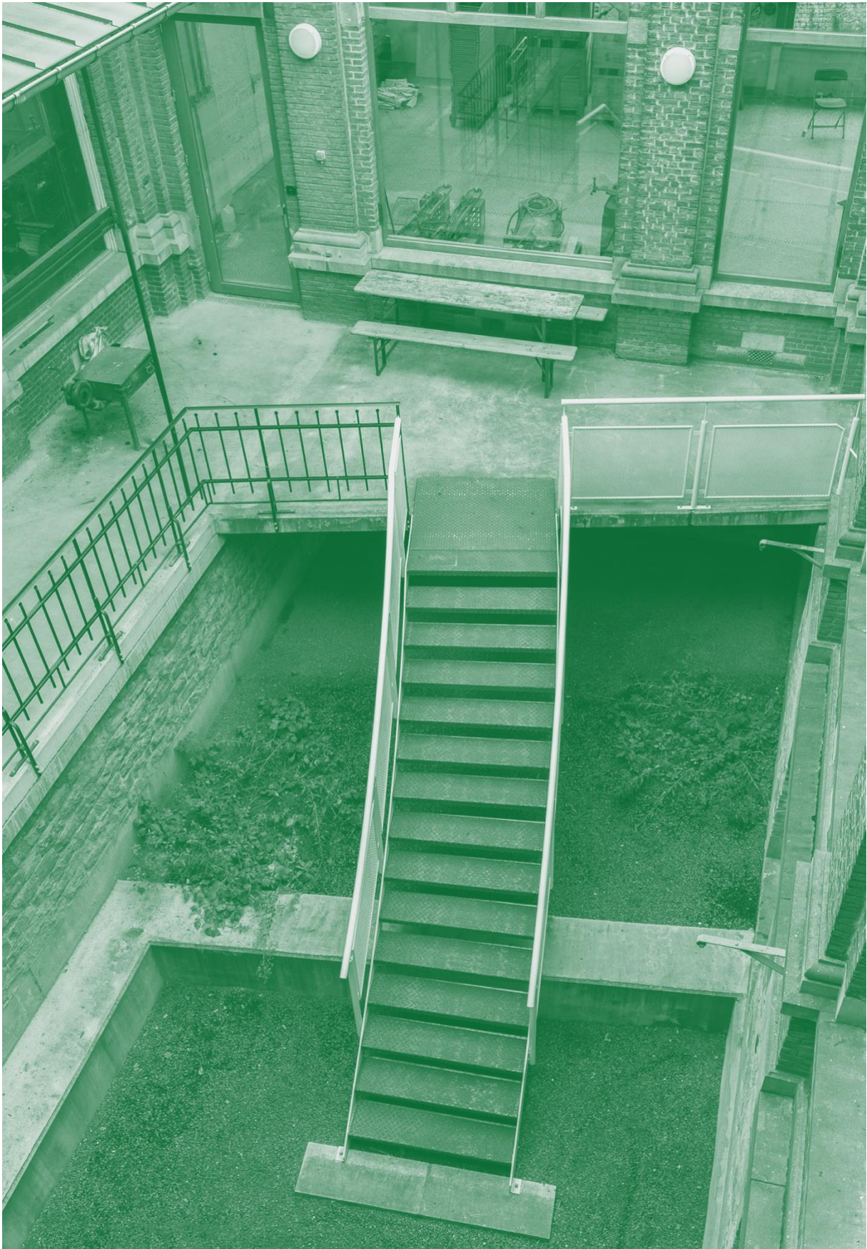
Figure 8: Reuse of a metal staircase by Rotor architects, Zinneke. Photo: Delphine Mathy.
