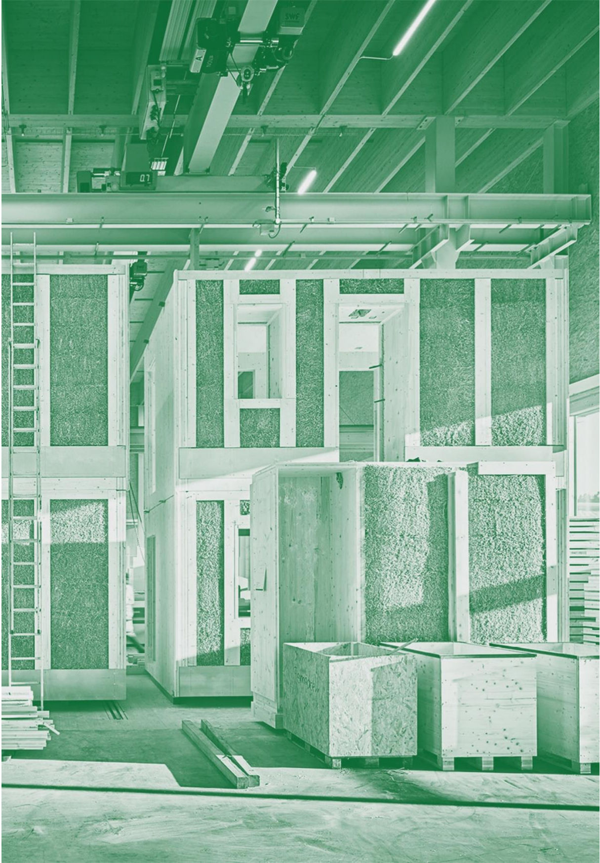
Figure 3: Wood wall panels with straw insulation, Bombasei. Photo: Unknown.
